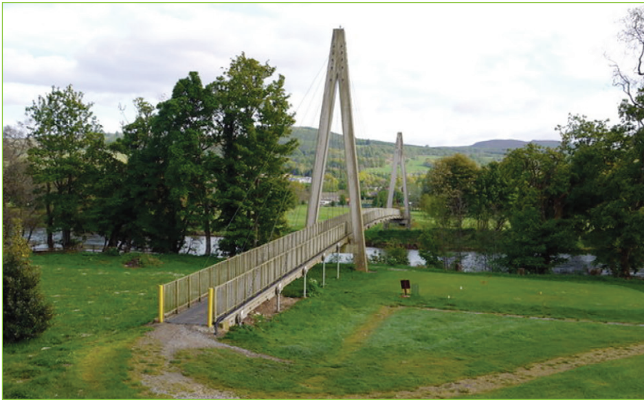
Fig. 2: Pedestrian bridge at the golf club in Aberfeldy (Scotland)
