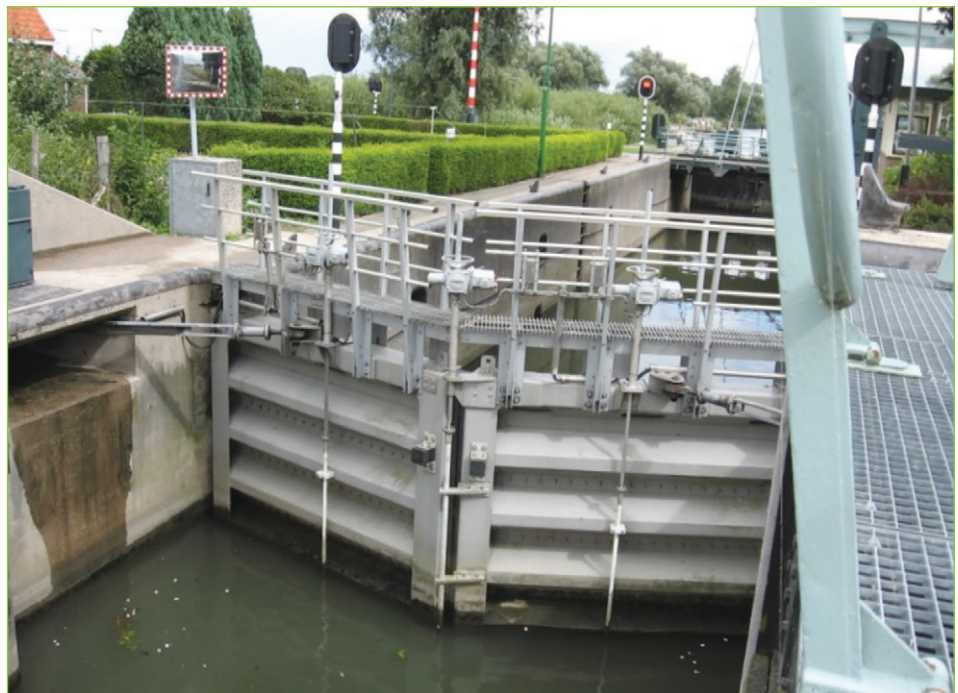
Fig. 1: Lock gate at Werkendam (Spieringsluis, the Netherlands)
