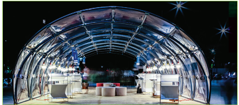
The TemporActive Pavilion, Politecnico di Milano. Construction materials by Top Glass Industries. [Courtesy of Top Glass Industries]
