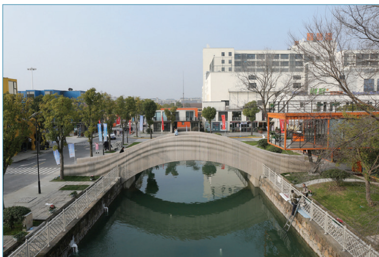
Fig. 1: The single-arch bridge structure was created using a 3D-printed concrete system developed by Professor Xu Weiguo's team (photo: Tsinghua University)
