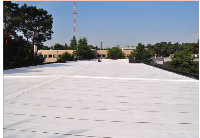
Reflective membranes on roof
