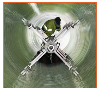
UV lamp curing a large diameter pipe
