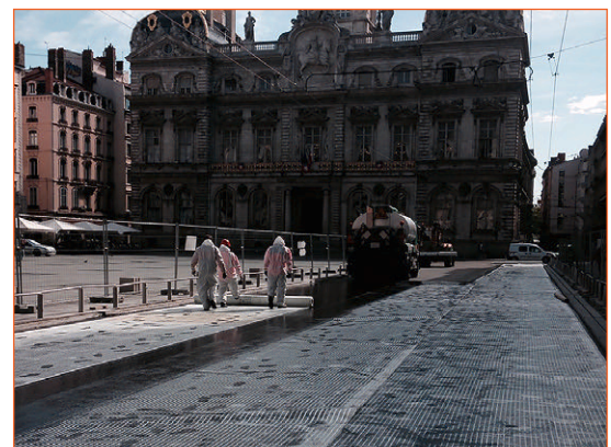
Glass fibre grid installed on road
