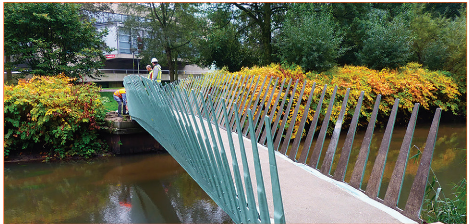
The world's first biocomposite bridge at Eindhoven University of Technology © archello
